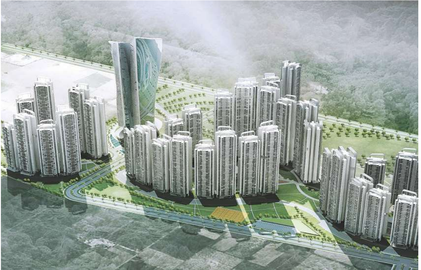
The Hues Mega Project, New Delhi, India Residential tunnel form system
